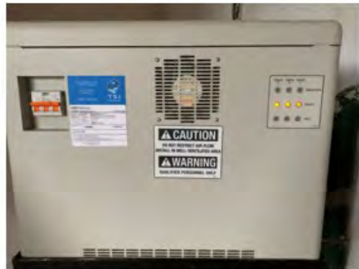
New Electrical Mainframe, Holding Ponds, and Pipeline at Salmon River Hatchery
